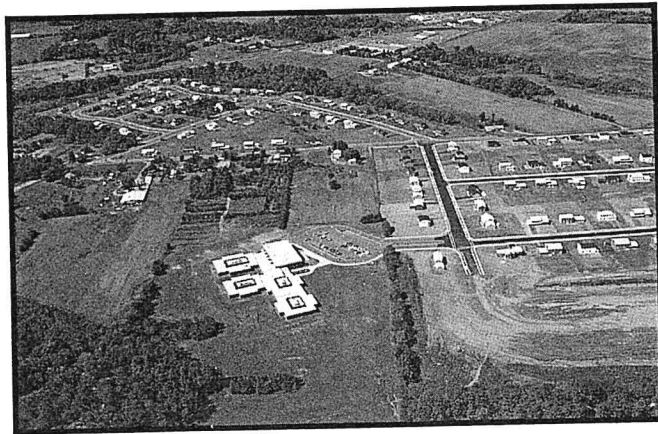
This image depicts a separation between residential and commercial uses making them accessible by car only. The positive feature of this image is the proximity to the school.
