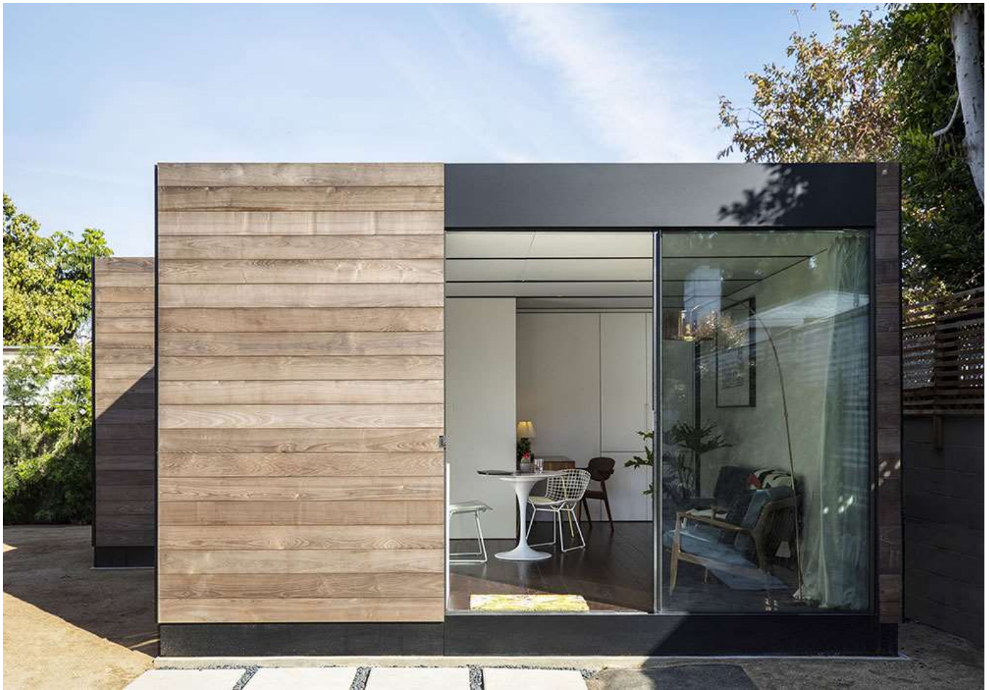
Los Angeles homeowners replaced their detached garage with this ADU created by local company Cover in 2019, three years after California allowed for ADUs in SFR zones. Photo courtesy cover.build (https://www.cover.build/) .
