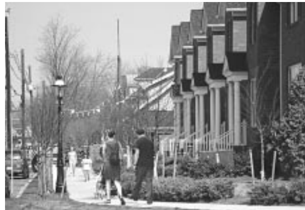
New infill housing located within walking distance of a train station supports transit and revitalizes communities.
