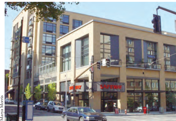
Figure 4.1.2. Mixed use zoning encourages pedestrian-oriented, storefront-style shopping streets that encourage physical activity and greater social interaction.
