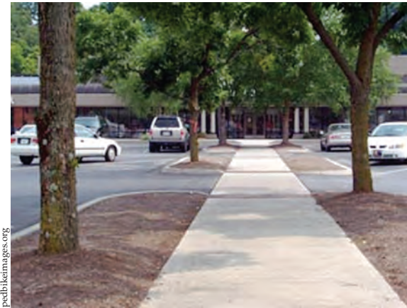
Figure 4.9.3. Walkways should provide easy pedestrian access through parking lots; this pedestrian walkway is clearly defined through the use of planters and alternate paving material.
