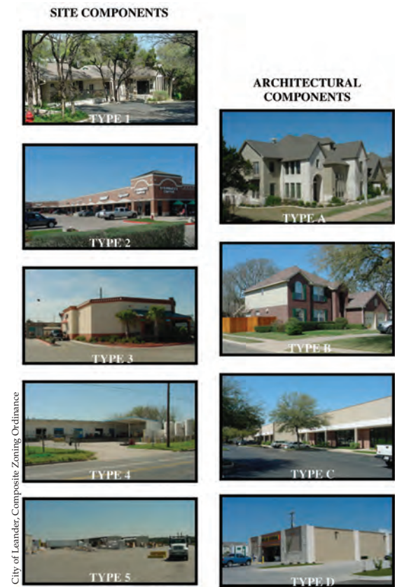
Figure 4.19.3. The composite zoning code of Leander, Texas provides five site components and four architectural components for developers to choose from.
