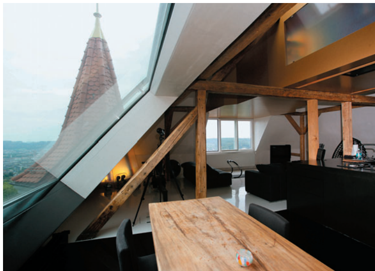
The structure of the house's old tower was cutting into the new living space, so Wüstemann created a negative space and then inserted a light sculpture into the cutout. The natural light that comes from the window of sloped ceiling augments the fireplace's glow.
